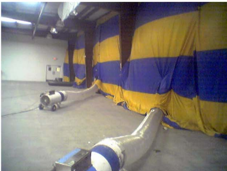
Insurers and property owners are finding that heat offers an effective alternative or adjunct to costly traditional demolition-based remediation and flood restoration.
